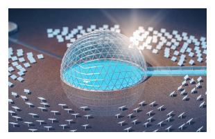
The solar dome project is a desalination plant that uses only solar energy to simulate the natural hydrological cycle process of evaporation, condensation, and precipitation. This technology employs a steel dome - a hydrological sphere – into which seawater flows. Solar radiation focused onto the steel frame using parabolic mirrors (heliostats) encircling the domes — the equivalent of up to 20,000 suns — provides the energy needed to superheat the constant supply of water
